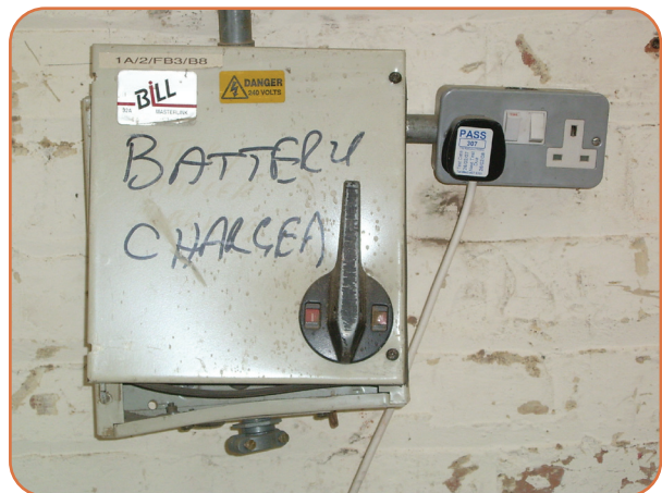
Figure 2-14: Defective electrical equipment. Source: FSTC Ltd.
